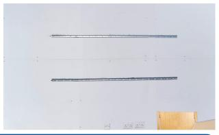
Next, install the glass board on to the rails, allowing the upper and lower clasps on the rear of the glass board to full engage and latch onto the rail.
